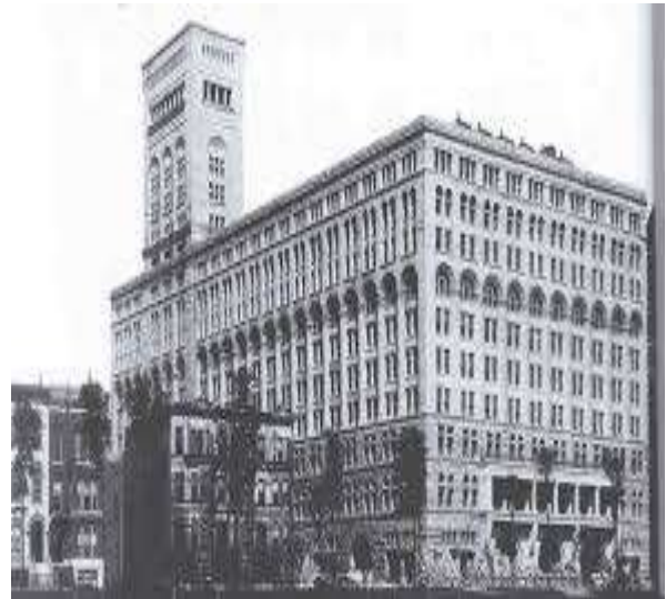
Figura 8. Sullivan Auditorium Building Chicago 1889.
